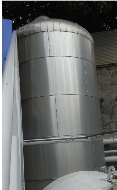
Figure 9. Buffer tank sitting outside the generation plant building
