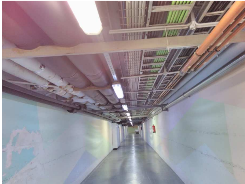
Figure 10. One of the underground galleries of the Hospital with the pipes of DC and DH installed in the ceiling (upper left corner)
