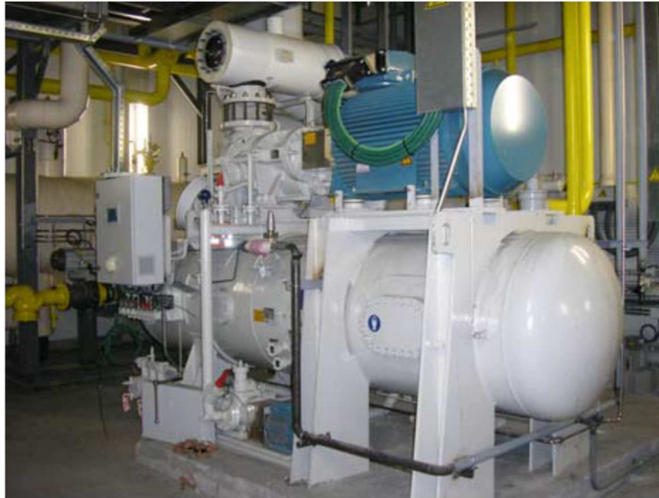
Figure 29. MYCON NV250 ammonia compressor
