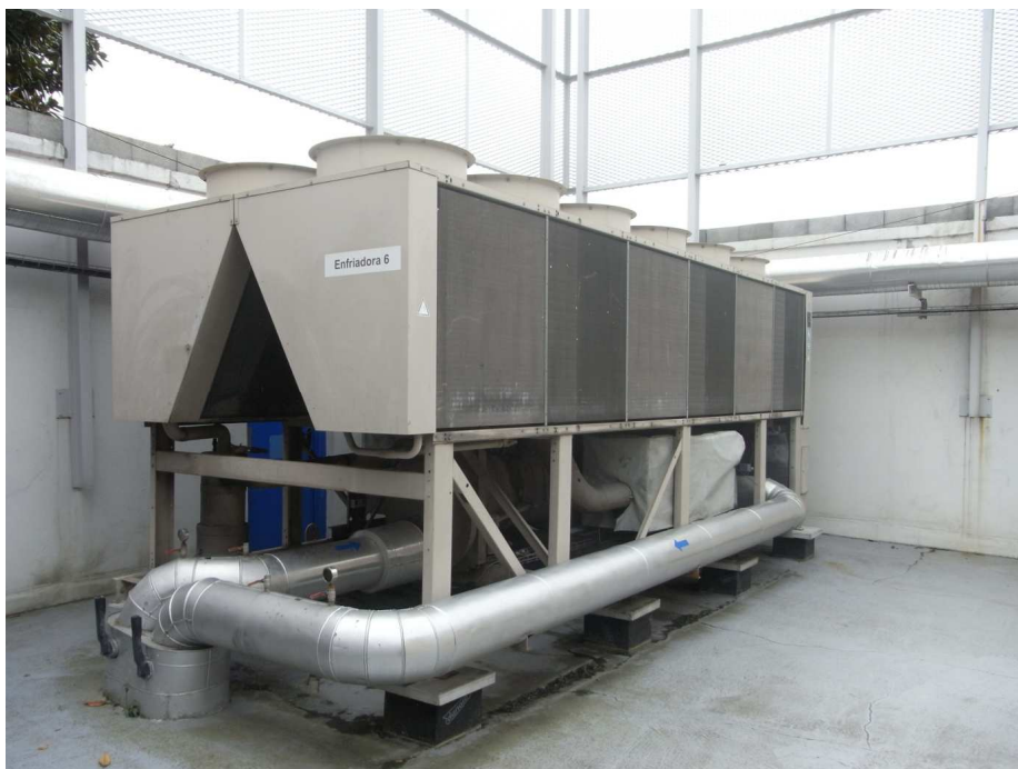
Figure 7. TRANE air cooled conventional chiller at its location in the roof of the generation plant
