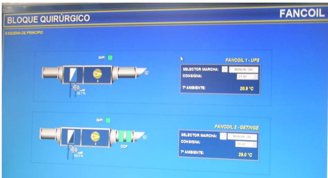
Figure 16. Screenshot from the BMS interface where two Fan coils installed in Areilza (Surgical Block) building can be seen in detail
