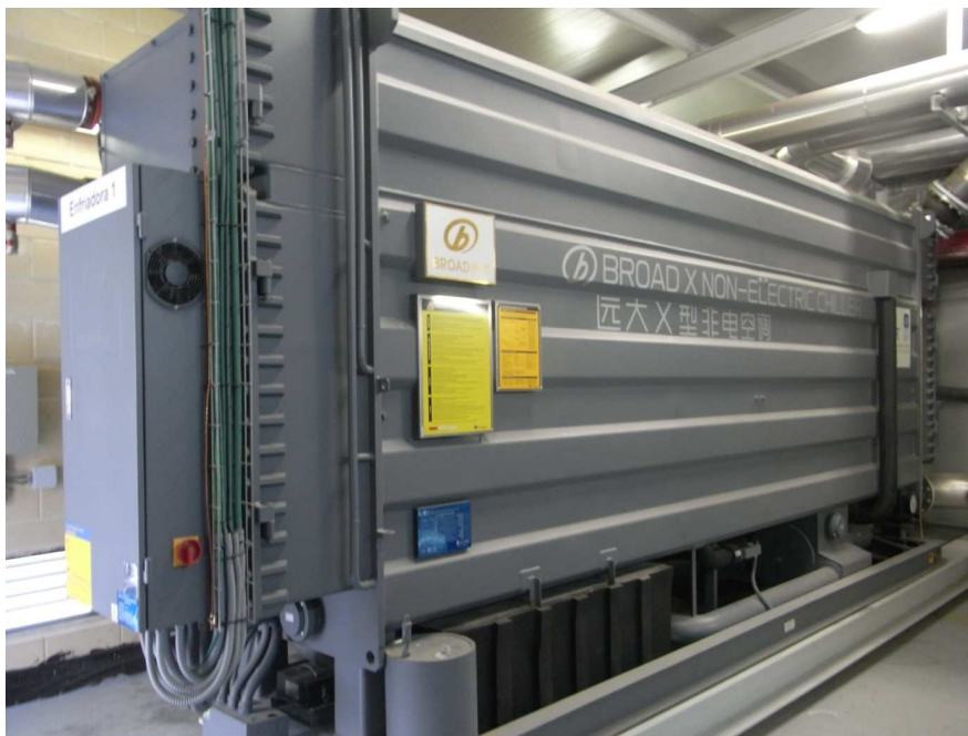
Figure 4. BROAD absorption chiller at its location in the generation plant
