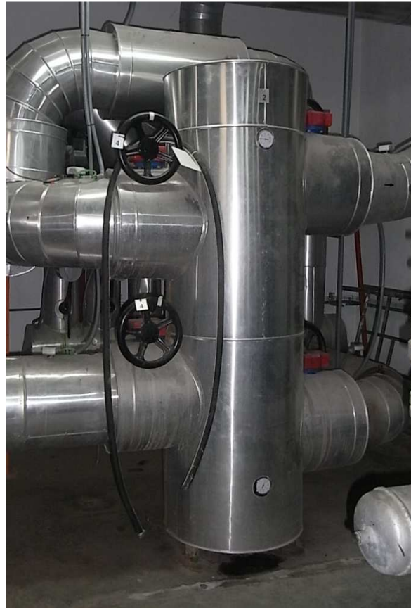
Figure 13. Hydraulic decoupler in one of the substations
