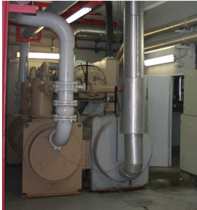
Figure 8. TRANE water cooled conventional chiller at its location in the generation plant
