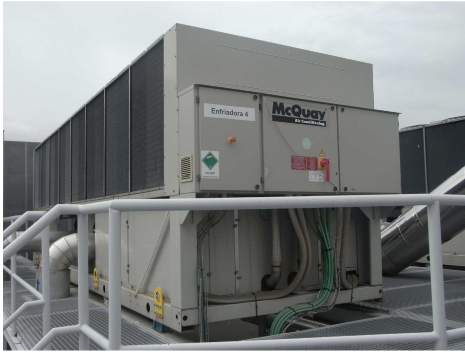
Figure 6. McQUAY conventional chiller at its location in the roof of the generation plant
