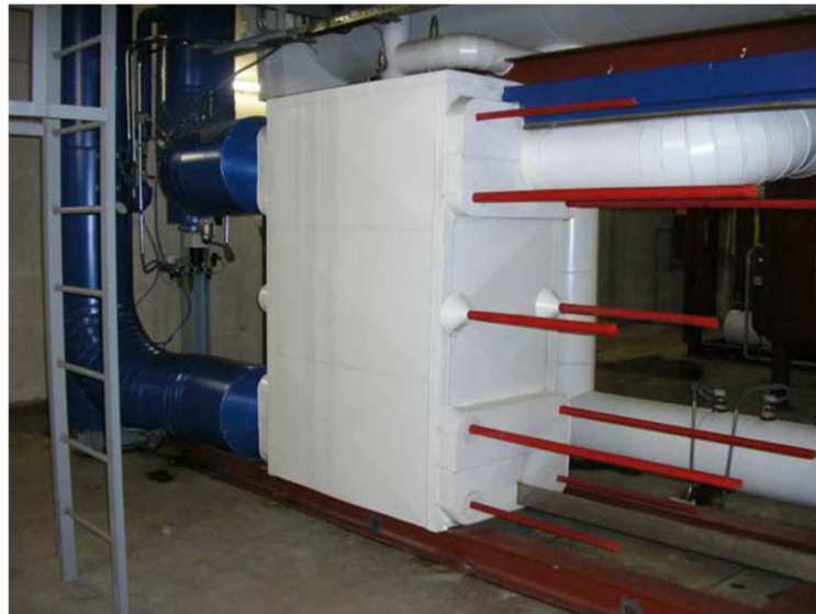
Figure 30. Flat plate heat exchanger for ammonia and water-propylenglycol mixture
